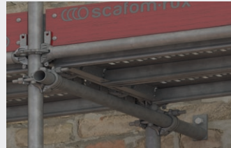
Figure 6.2c: Example of a tie bar test
